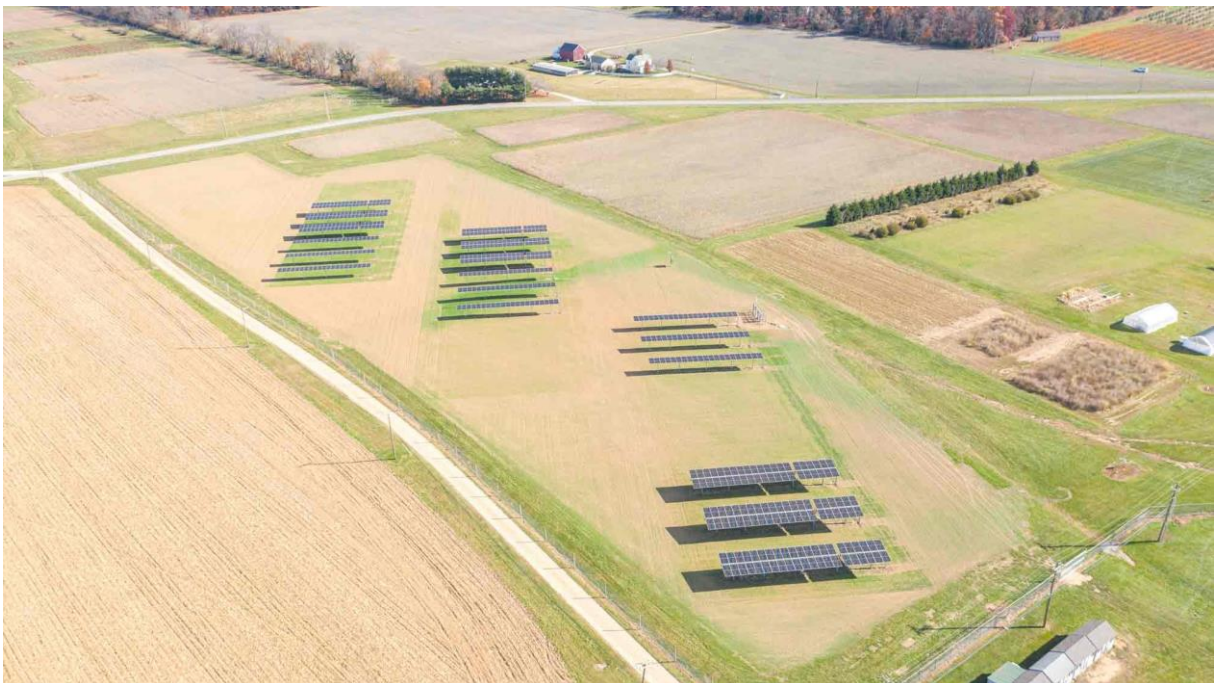
Figure 2. Rutgers Agricultural Research and Extension Center, Upper Deerfield, NJ ( 255\text{ kW}_{\text{DC}} installed, 48.6\text{ kW}_{\text{DC}} grid-connected, single-axis trackers with a pivot point 2.44 m (8 feet) above ground level): Staple and specialty crop production. Three randomized blocks, each with a control area, three rows with single rows of panels, and three rows with double rows of panels. Row spacing: 10.36 m (34 feet). Each North-South-oriented row has either 21 or 42 bifacial panels. Drone image taken looking toward the East (image courtesy of Advanced Solar Products).
