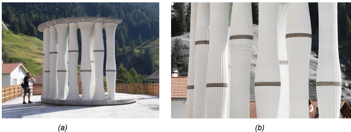
Figure 2. Demonstrator assembly with dry connections: (a) ten columns and two precast slabs are post-tensioned with steel rods; (b) detail of the assembly connection with the precast elements, images: Hansmeyer/Dillenburger.
