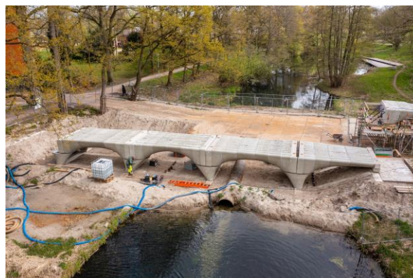
Figure 8. Assembly of the final bridge on location
