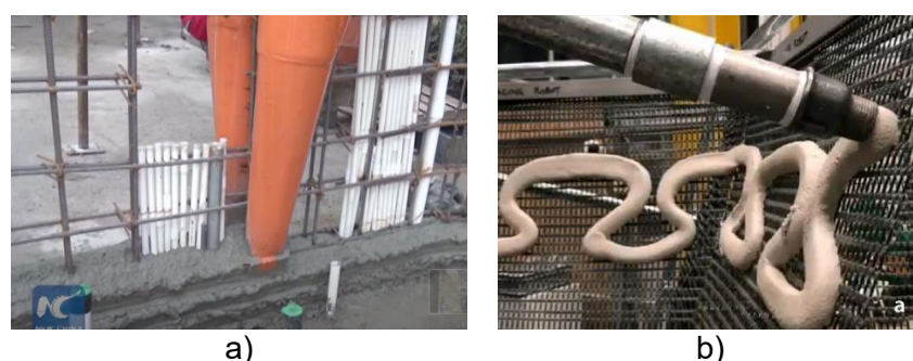
Figure 1. Introduction of reinforcement prior concrete printing: a) 3D printing around the steel meshes using bifurcated printhead [17] and b) extrusion-based material deposition on a fine textile mesh [18].
