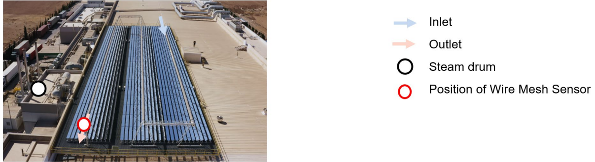
Figure 1. Bird's eye view of the Fresnel solar system (Photo: Industrial Solar GmbH)
