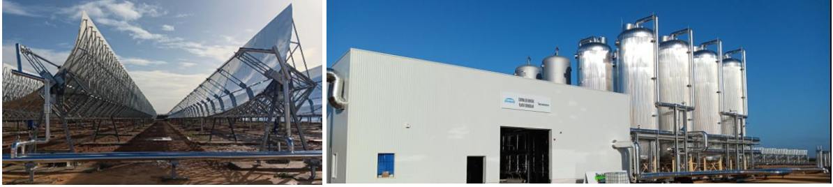
Figure 6. Left: Solar collectors at Heineken plant in Sevilla operated by ENGIE (Source DLR), Right: Balance of plant and 8 storage tanks (Source DLR)
