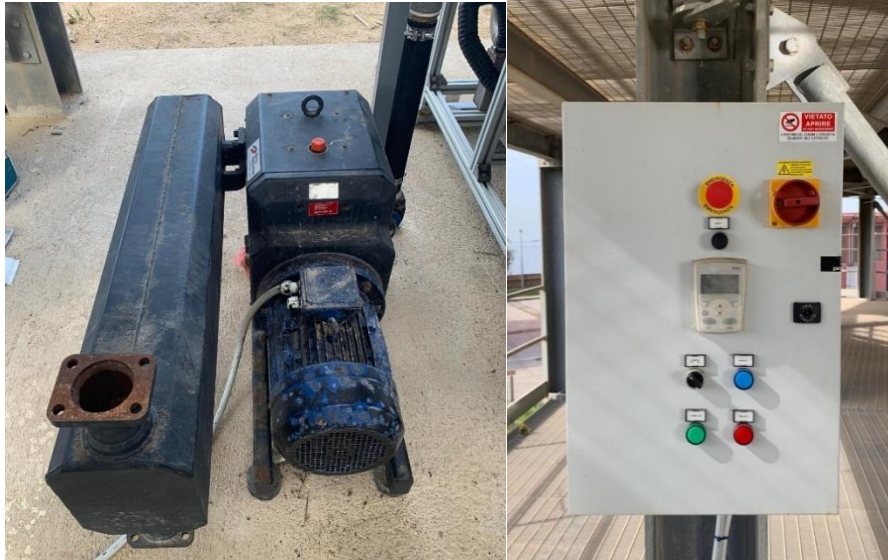
Figure 3. 7.5kW air compressor and its control box mounted in the plant
