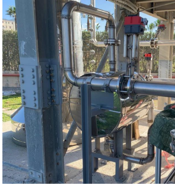
Figure 4. Heat recovery unit installed in thermal plant
