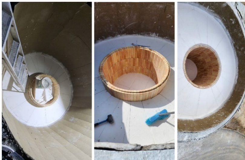
Figure 3. Construction progress of the HDFB and Ca-Si layers
