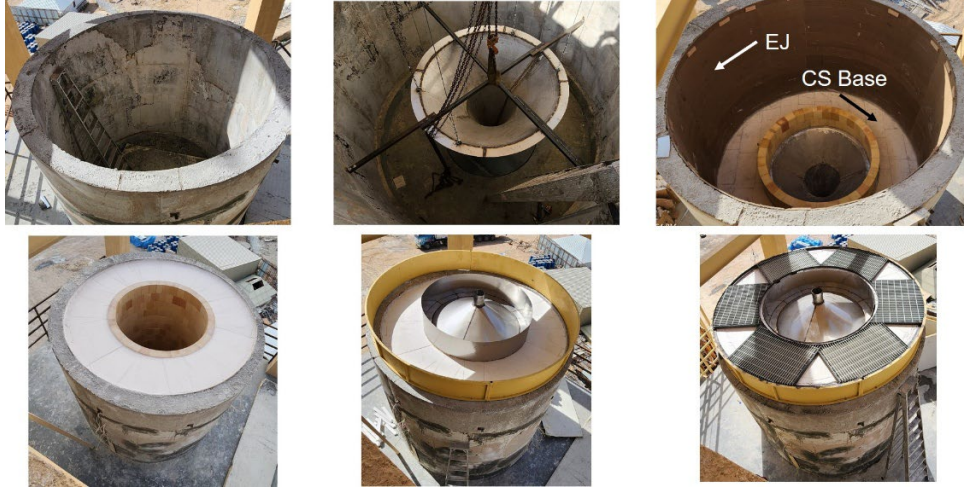
Figure 7. Construction stages of the near-scale TES bin
