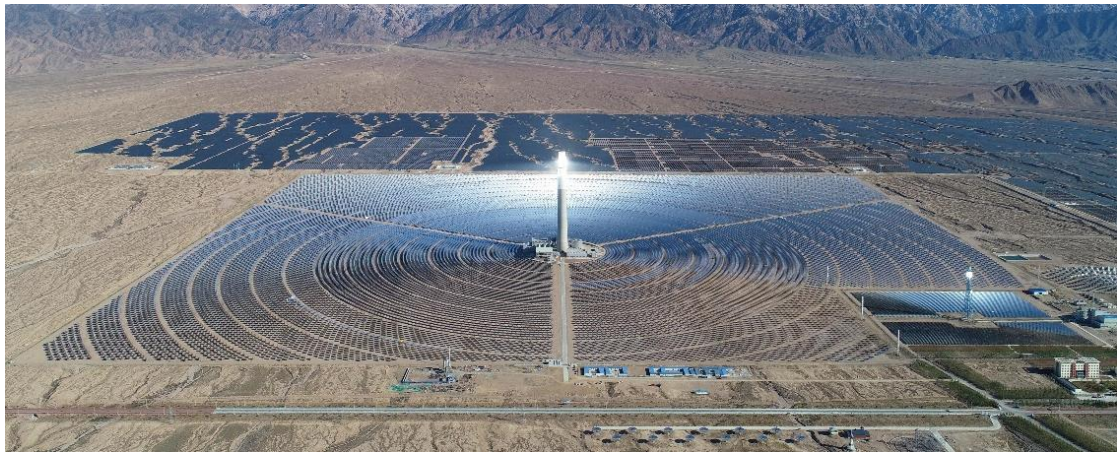
Figure 1. Panorama view of SUPCON Delingha 50 MW CSP station (Zhejiang SUPCON)
